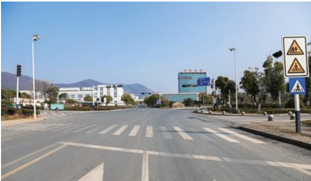
为五岔路口安装红绿灯
